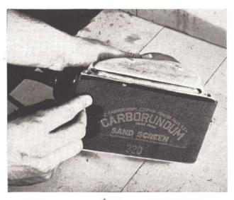
Sandpaper takes a new form. Residue won't clog mesh, which has an abrasive coating on both sides.
